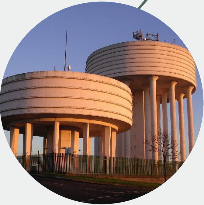
GARTHAMLOCK AND CRAIGEND WATER TOWERS
